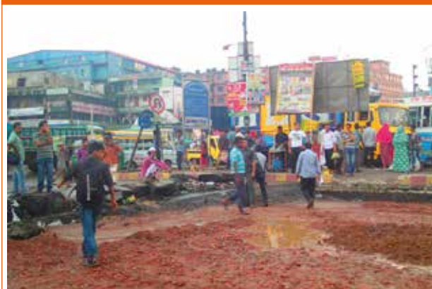
Picture 4. Road between Dhaka and Chittagong
